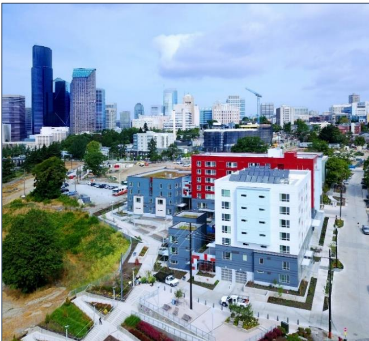
An aerial view of the newly constructed Hoa Mai Gardens, showcasing the solar panels and green roofs.
