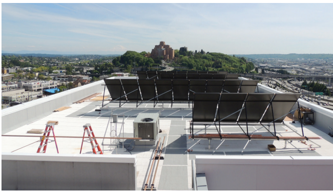
Figure 5: Solar hot water systems at Lake City Court (top) and solar panels at Hoa Mai Gardens (bottom)
